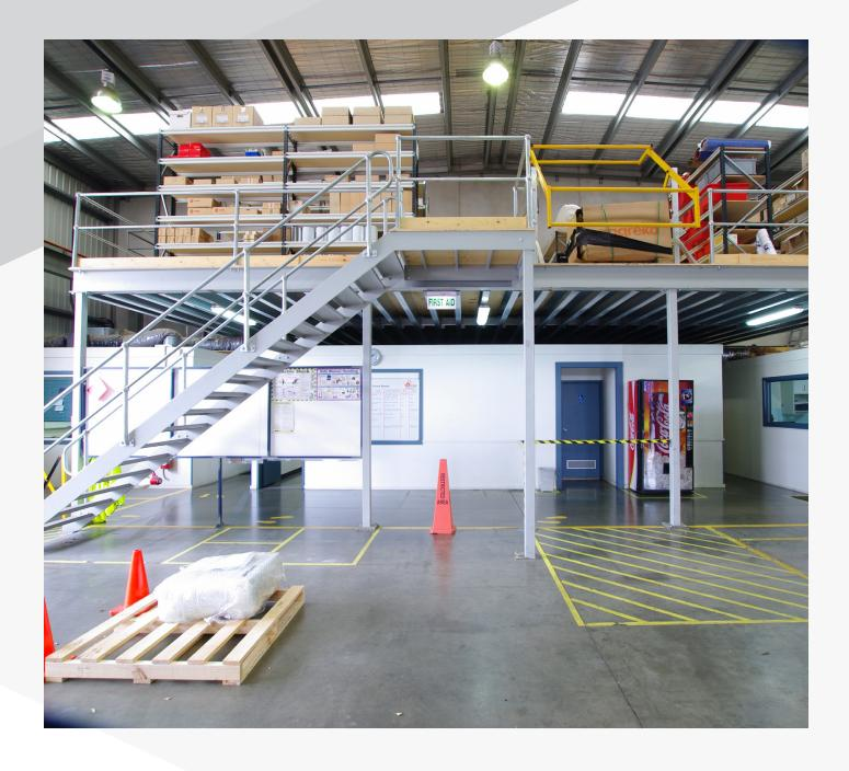
Mezzanine floor main support beams can be built to any specification. Your mezzanine floors unique loading requirements determine the thickness of the beam and the spacing required between columns.
